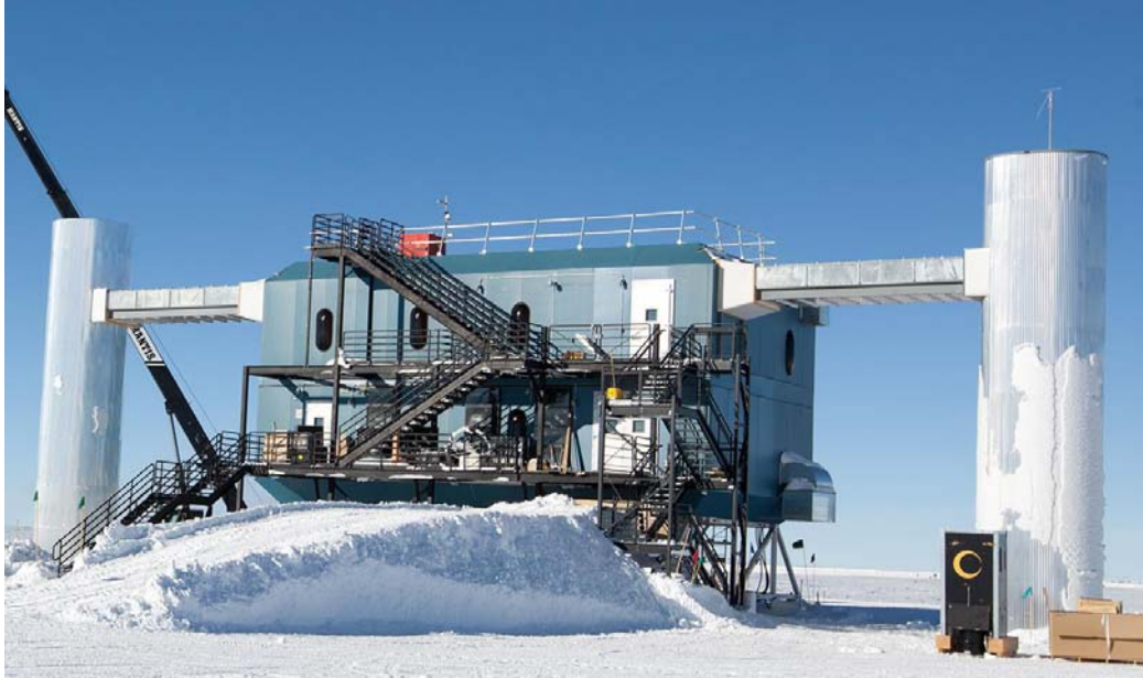
Figure 3.2-1. IceCube Laboratory (ICL). The ICL at the South Pole houses the online computing system which is critical to mining data from IceCube.
